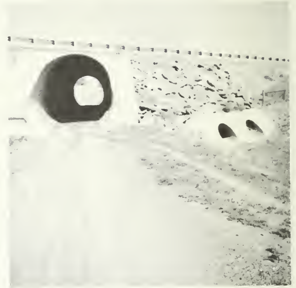
SOUTH ENTRANCE; Notice drainage pipes
